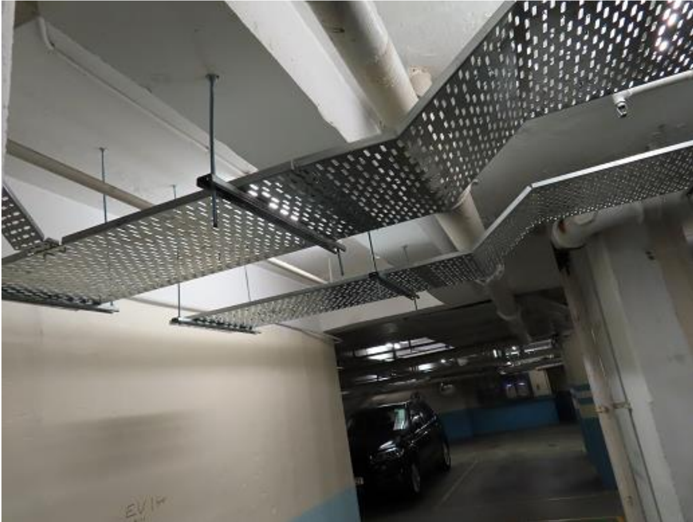
Installation of cable containments in the car park
